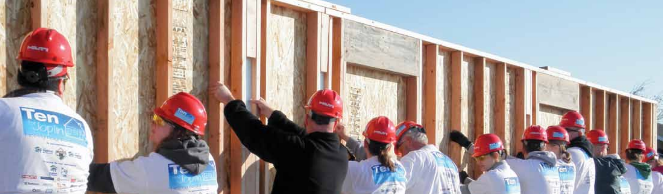
BKDer's raise a wall during the Ten for Joplin blitz build
